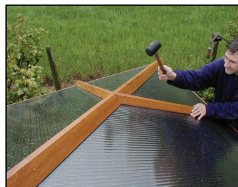
4) All glazing can now be carried out. When fitting the Top Caps, ensure that the Joint between the Hip Top Cap and the Jack Rafter Top Cap is sound.
