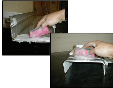
2) Smear soapy water on the inside face of the Box Gutter where the Adaptor will locate and to the seal that is fitted on the Adaptor.
